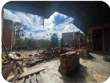
our new construction site
