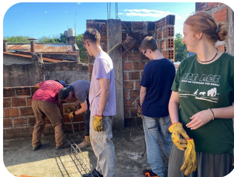
Getting a frame for the roof ready
